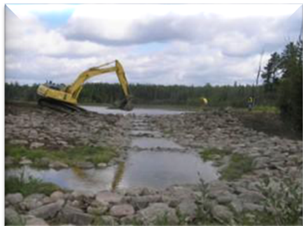
The newly created channel.
